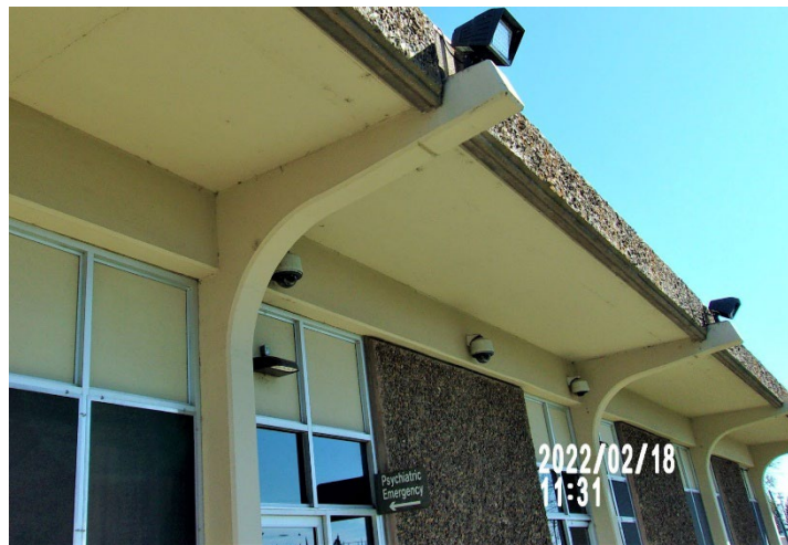
(Cameras at the entrance of the Psychiatric Health Facility were poorly spaced, which provided inadequate coverage.)
