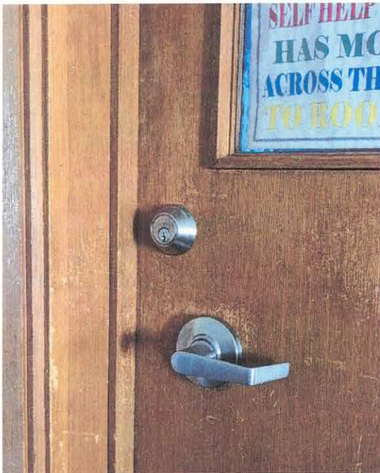
Photo 3: Deadbolt lock on interior door to the Grand Jury room.
