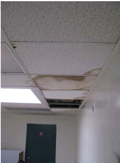
Water damage to ceiling
