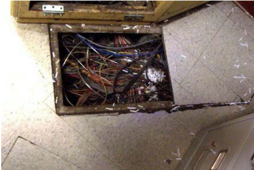
Exposed Wires on Floor of Control Room
